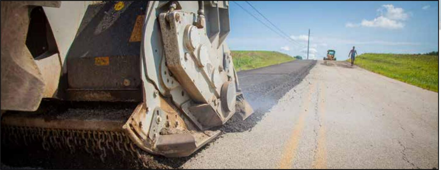
The department's 13,448-lb. FAE MTM 225 is a versatile, all-in-one soil stabilizer, rock shredder, stone crusher and asphalt shredder. The 225 grinds to 16" and pulverizes to less than 3/4", grinding as well as a milling machine according to Christopher Young. The reclaimer offers a variable shredding chamber requiring tractors between 240 and 360 HP.
